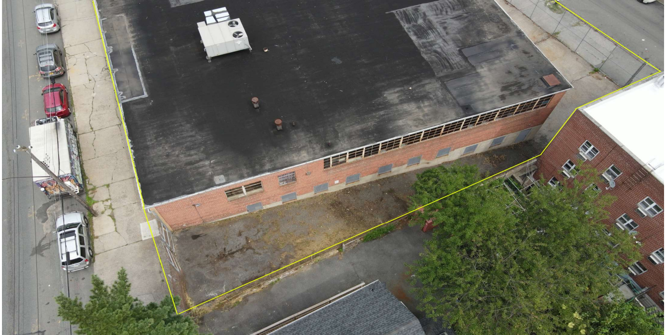
South to North View of the driveway
