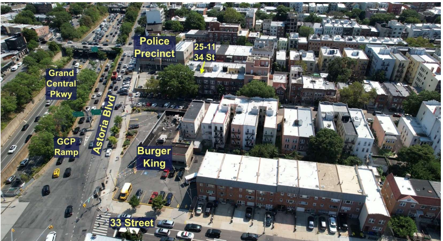
West to East Aerial View
