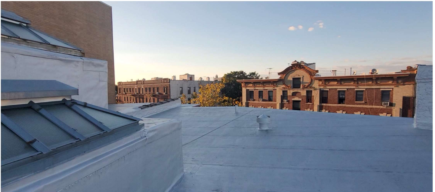
ROOF REAR AND SIDE FACING FARRAGUTH ROAD
