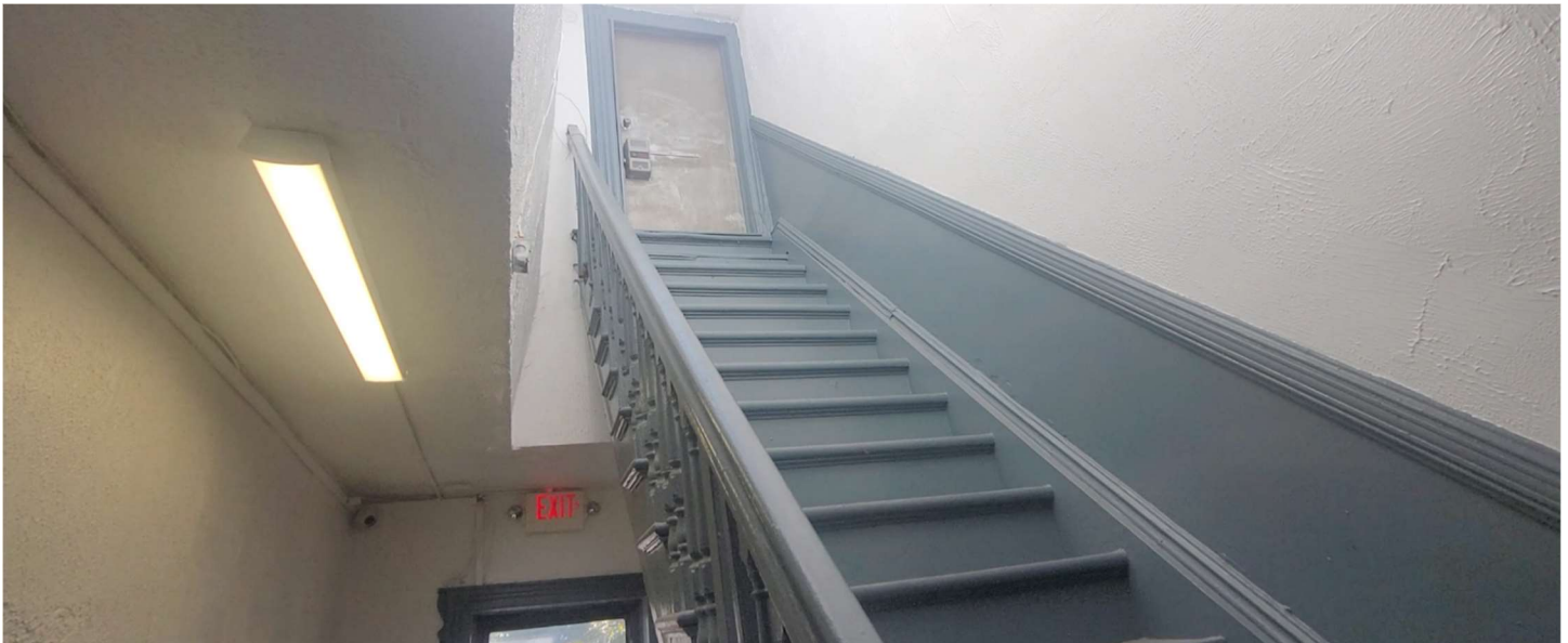
STAIRWAY TO ROOF AND SKYLIGHT
