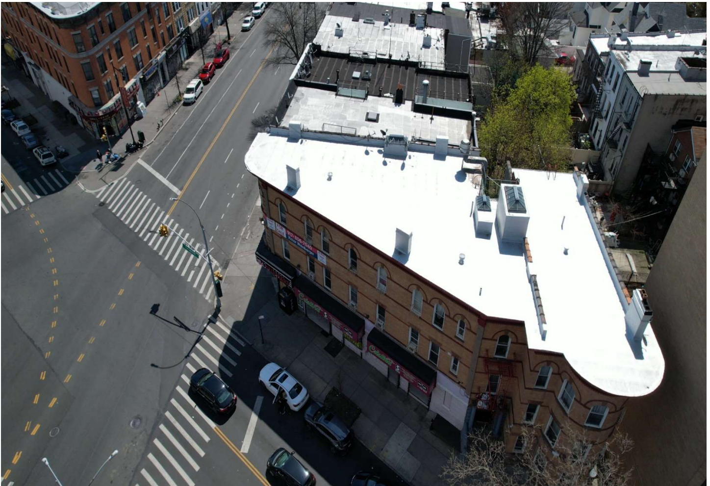
BUILDING ROOF VIEW UP CLOSE
